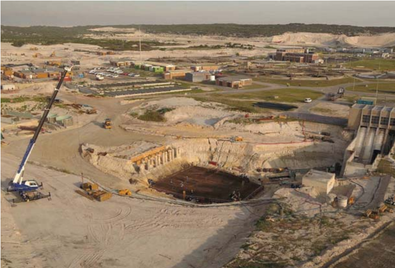
Waste not, want not: The upgrade to the Zandvliet wastewater treatment works will create additional capacity and produce cleaner discharge.
